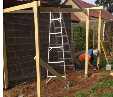
New woodshed construction at the hall
